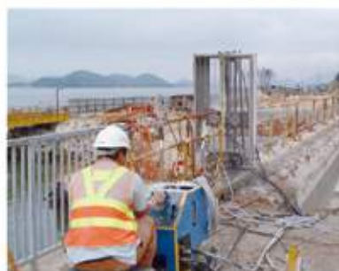
Wire Sawing 鑽石鏈割
