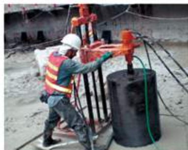
Diamond Coring 鑽孔
