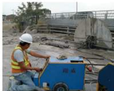
Wall Sawing (1000mm deep) 牆割 (厚一米)
