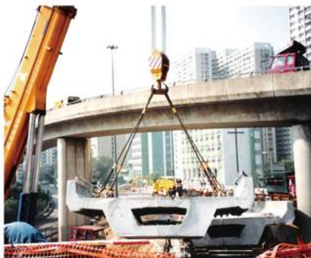
Footbridge Demolition 拆卸天橋
